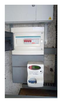
Other pictures that detail the structure of the intervention. The first one is the main electric panel, equipped by the POD and 1 smart meter for the energy metering of 1 staircase.
